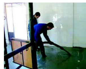
4. Self levelling application
